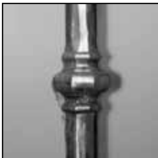
Example of a stainless steel picket polluted by external agents like dust and smog
